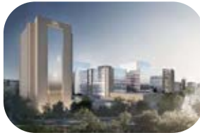
HOSPITAL ÁNGELES DEL PEDREGAL CDMX
